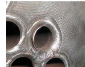
The use of a hydraulic expander provides a more uniform expansion and superior contact of the sleeve OD with the ID of the parent tube. Additionally, the sleeves were strength welded to the parent tubes at the face of the outlet tubesheet
